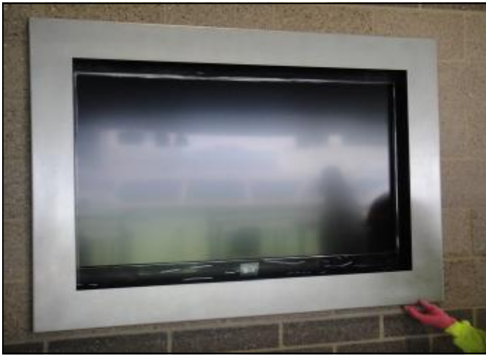
Enclosures for 55 inch televisions on the Concourse Level
