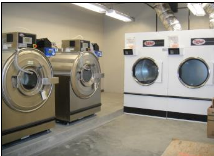
Installation of washers and dryers
