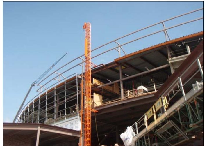
Installation of glass wall framing behind home plate
