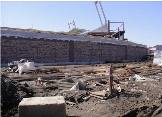
Forming of concrete walls for field material storage
