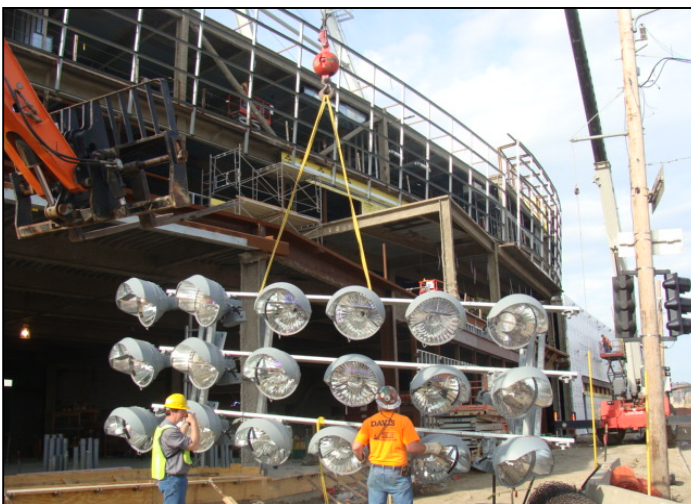
Installation of sports lights on the left field tower
