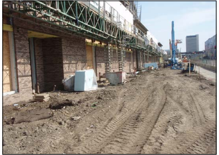
Installation of brick along 13th Street
