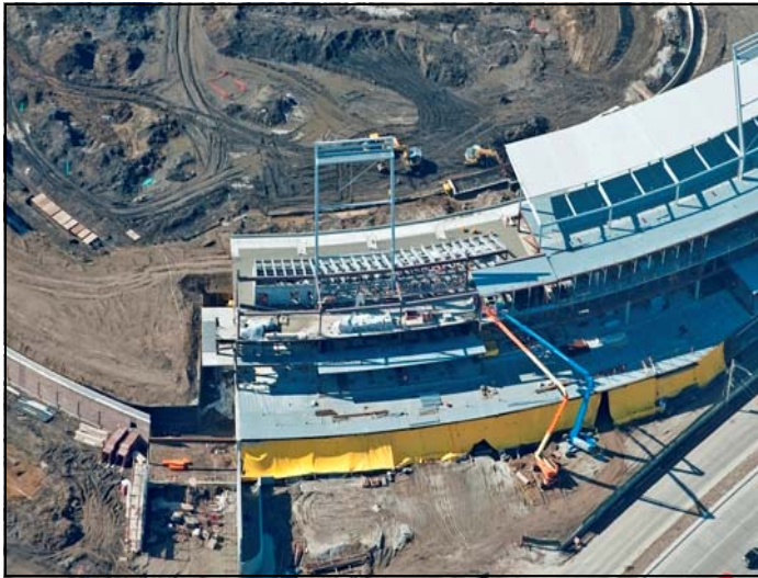
Installation of the curtain wall framing at Cuming Street
