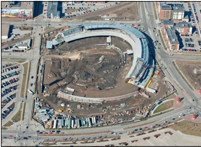
Aerial view from 10th Street
