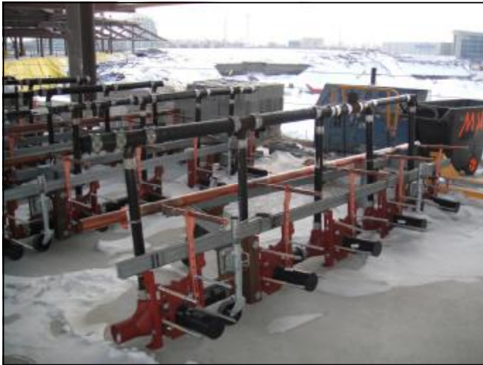
Pre-assembled restroom plumbing piping
