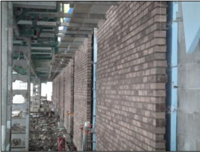
Installation of exterior brick and block walls
