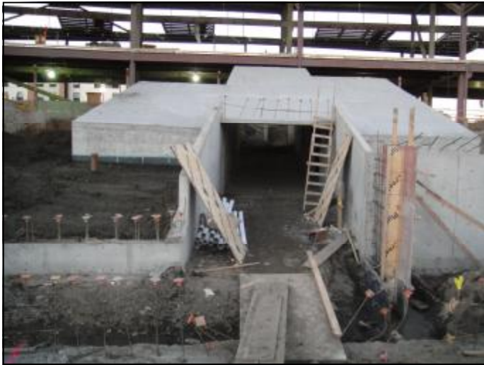
Field access tunnel along 1st base
