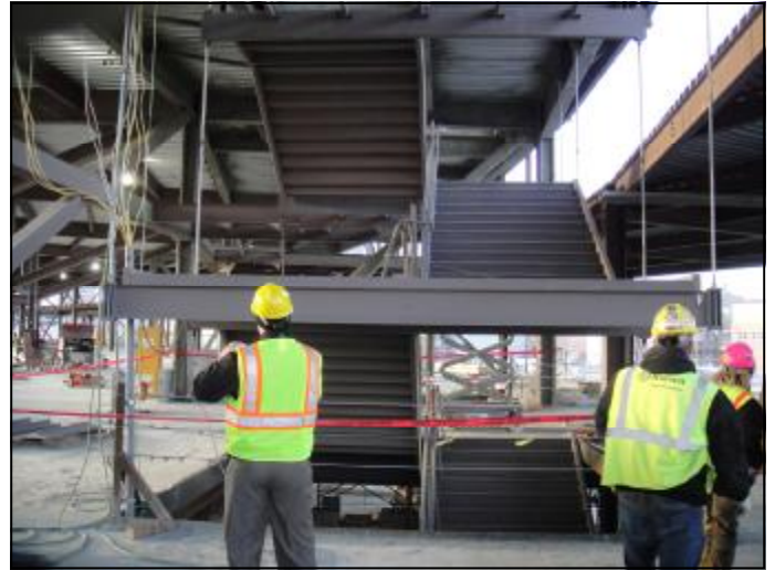
Interior stairs construction
