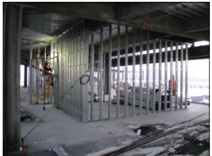
Installation of Suite Level metal stud walls
