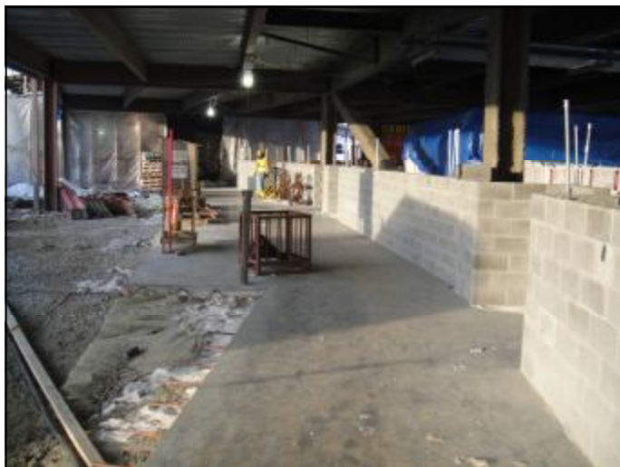
Installation of interior concrete block walls
