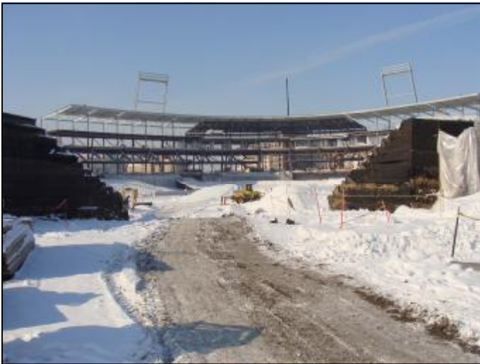
View of stadium from outfield access area
