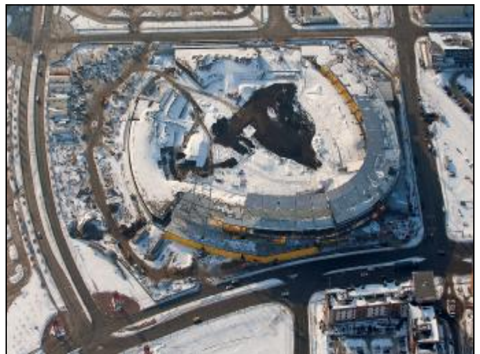
Aerial view of the entire construction site
