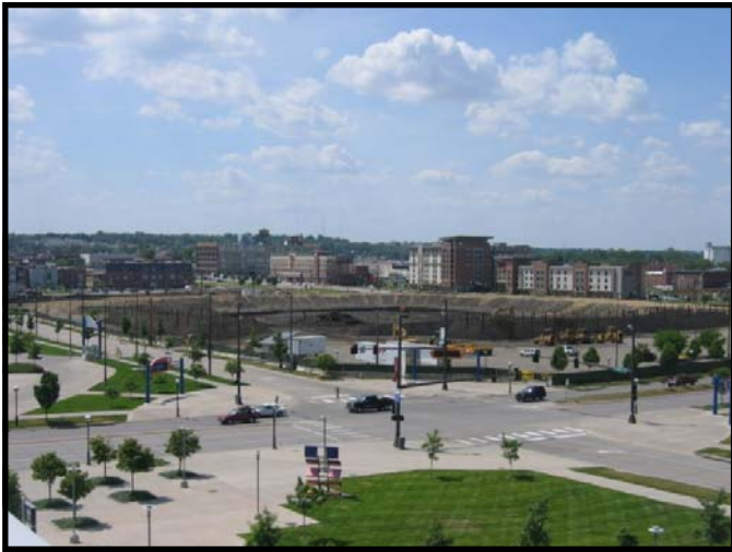
Stadium site looking northwest
