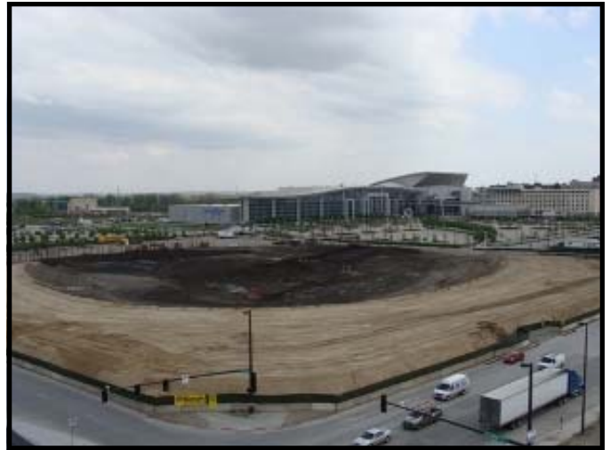
Stadium site looking southeast
