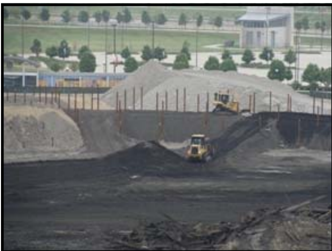
Adding soil surcharge to outfield areas
