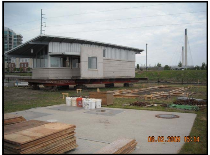
New foundation formwork for the Parking Control Center
