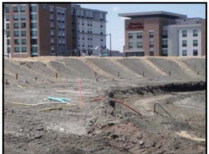
Removal of soil down to playing field level
