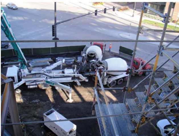
Concrete operation for placement of concrete on Main Concourse
