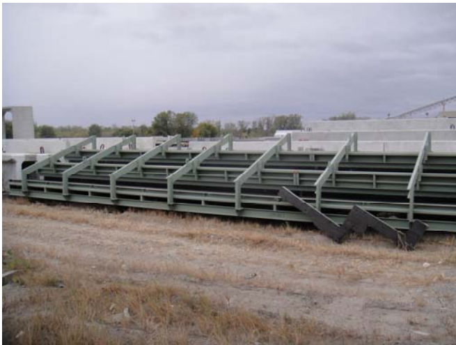
Steel structures to form Club Seating risers
