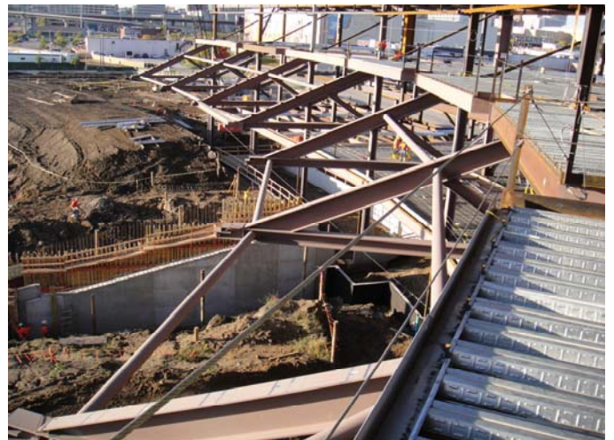
Steel to support the concrete precast risers on Suite/Club Level
