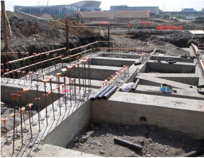
Concrete footings for tunnel access to the Playing Field
