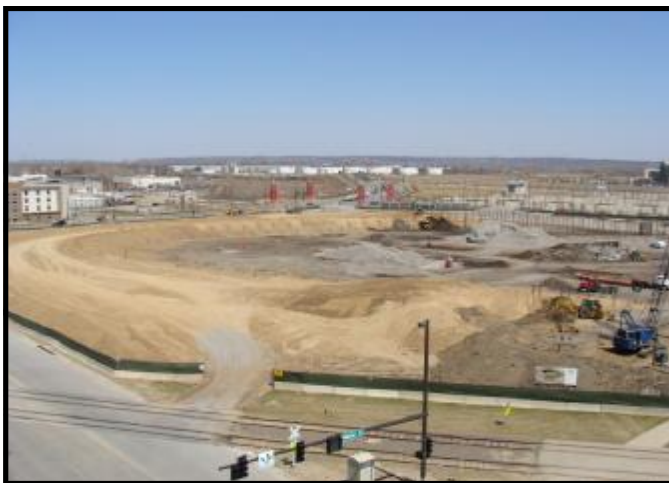
Stadium site looking northeast
