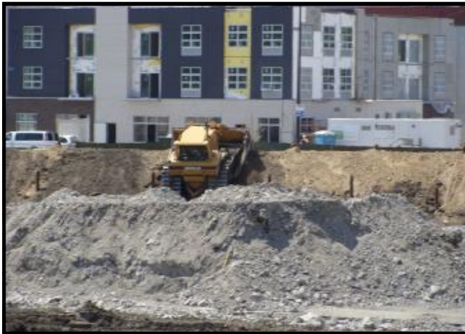
Placing surcharge to form the concourse and seating bowl areas
