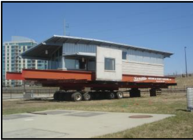
Parking control building temporarily moved to the new location
