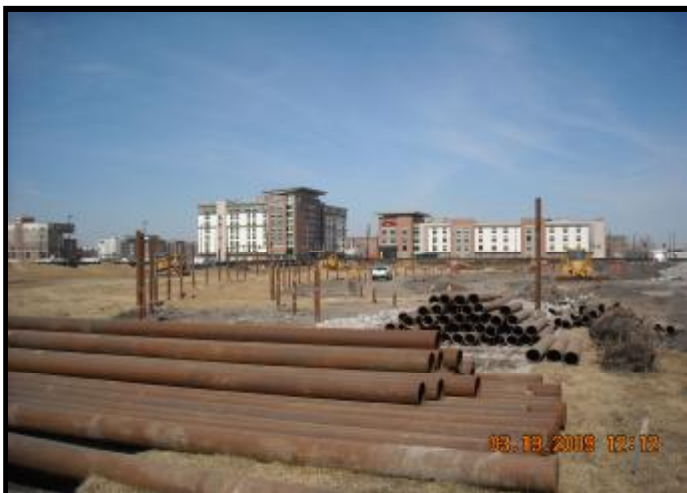
Piling for Seating Behind Home Plate and along First Base
