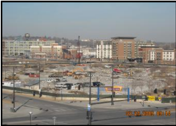
Demolition Work Continues
