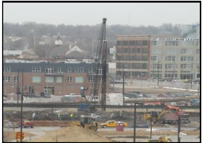
Piling being Driven at Concourse Areas to be Supported by Surcharge
