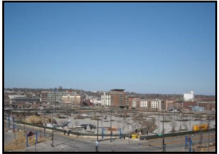
Demolition Work Begins by Crushing Concrete Paving Areas
