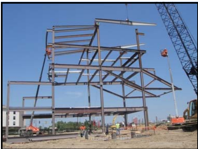
Steel being installed to form the building structure behind home plate
