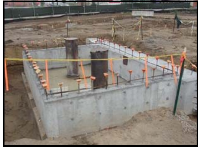
Concrete base of the tower for the media elevator
