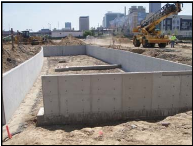
Concrete walls of the batting tunnel along the 1st base line
