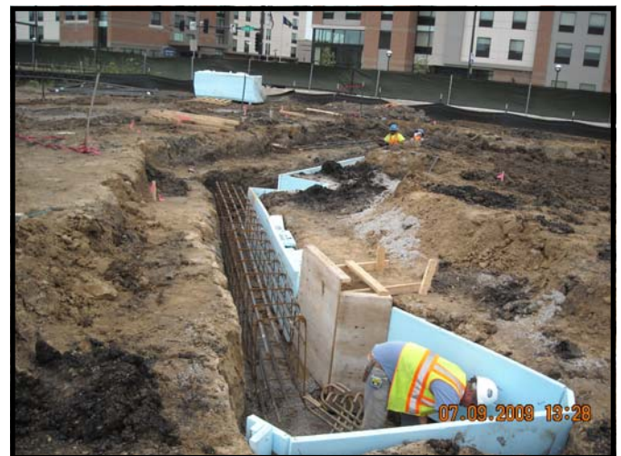
Placement of forms for the perimeter foundations around the building
